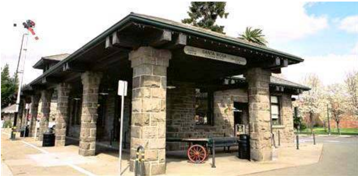
The location can be found at the Railroad Square in the old Train Depot building.
