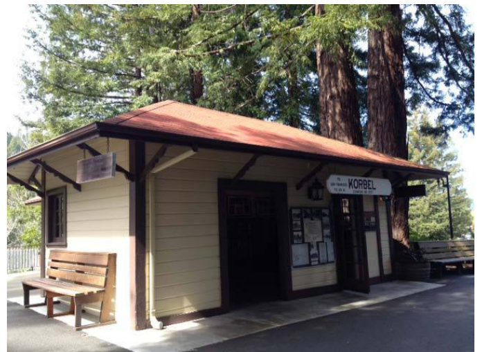
Satellite location in the Old Train Depot.
